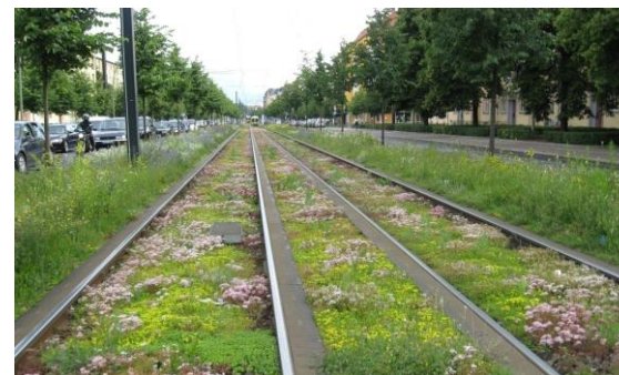
Figure 16 A tram track vegetated with Sedum plants in Berlin.
