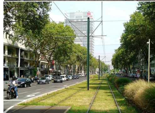
Figure 18 The same tram track in Düsseldorf after greening.
