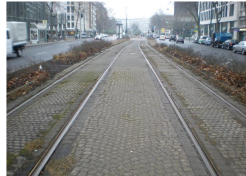
Figure 17 A tram track in Düsseldorf before greening.
