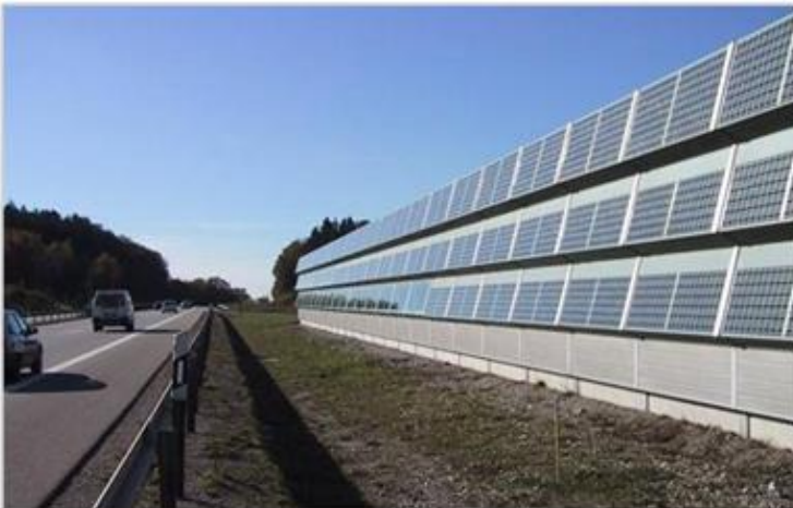
Figure 36 Solar panels on a noise wall in Germany.
