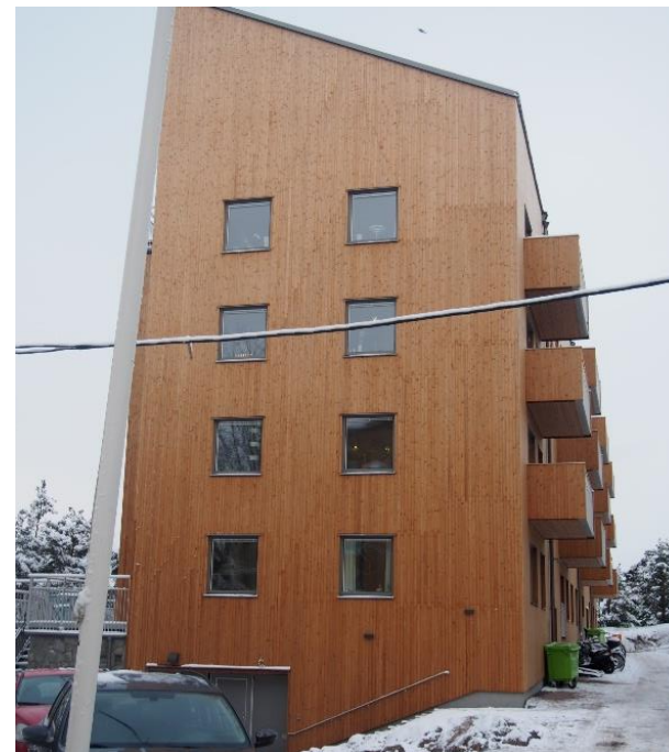
FIGURE 1. WOODEN FAÇADE ON NEWLY BUILT RENTAL HOUSING (TAKLAMPAN) CLOSE TO HAMMARBYSKOGEN (FINN MALMGRENS VÄG). HOUSES ARE CLASSIFIED AS ZERO ENERGY BUILDINGS AND CONSTRUCTED TO SAVE ENERGY THROUGH LOW HEAT LOSS. SOLAR PANELS ARE PLACED ON THE ROOFS TO COMPENSATE FOR ENERGY USAGE. EINAR MATTSSON.
